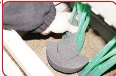
**Step 4** – Make sure each duct has the foam pushed in leaving a 20mm space at the top.
