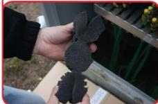
**Step 3** – Push the foam into the duct ensuring the centre pieces of the foam is in the centre of the micro ducts. The foam will then sit nicely around all the tubes.
