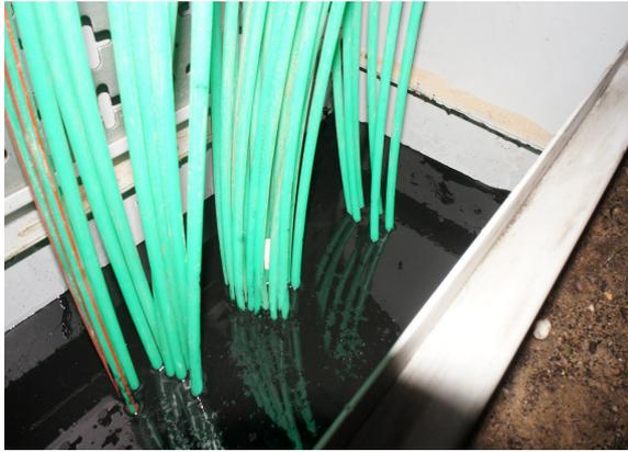
2 component sealant used to seal the base & ducts in Virgin Media's street cabinets.
