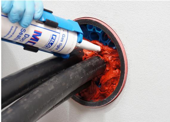
Duct sealing system FiloSeal+HD is an engineered universal solution for sealing larger heavy cables and pipes in ducts, boreholes or transit frames.
